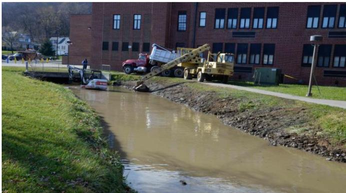
After a phone call and a couple of emails, it was determined that the firm doing the excavation had a permit to do the work, and that the use of hay bales was in compliance with permit requirements. A West Virginia DEP official later noted that the bales work fine if properly placed, but that they should not have been placed in a riffle.
